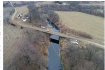
Emergency crews work to clean up the largest U.S. crude oil spill in nearly a decade, following the leak at the pipeline operated by TC Energy in rural Washington County, Kansas
